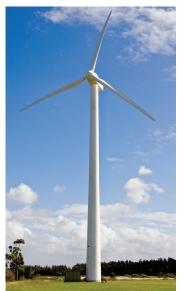
Wind power is harnessed by installing wind turbines which in turn can be used to generate electricity for use in homes and businesses. Wind hits the blades of the wind turbines, causing the blades to turn. This movement drives a generator which produces electricity.
